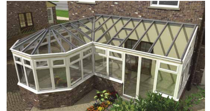
The aluminium rafters, ridges and wall plates are fitted and the spider arms are secured to the spider bracket.
